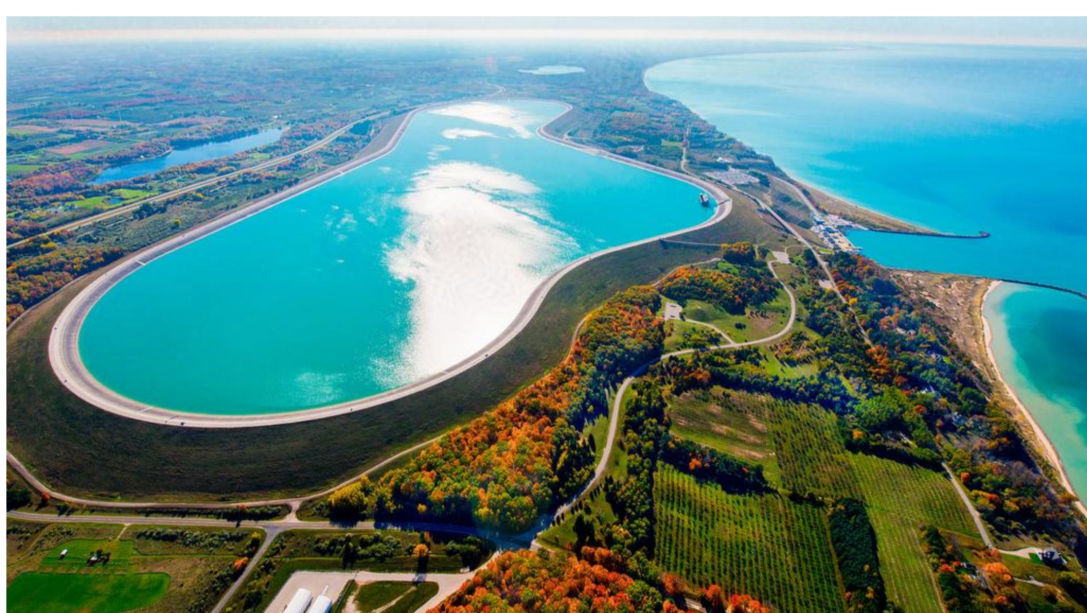
Aerial picture of the Ludington Pumped Storage Facility [3].
